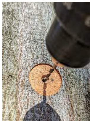
2.6.2 Prepare a 4 cm deep hole with a 4 mm drill bit.
