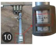
Checking the tightness of the M10 screws in CBS Anchors (= 40 N\*m).
