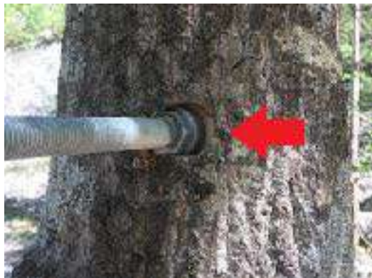
Photo taken during pull-out test on the Anchor Nail
