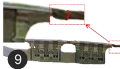
9 Checking cable displacements at the beginning and end of Double Arms intended for ziplines.
