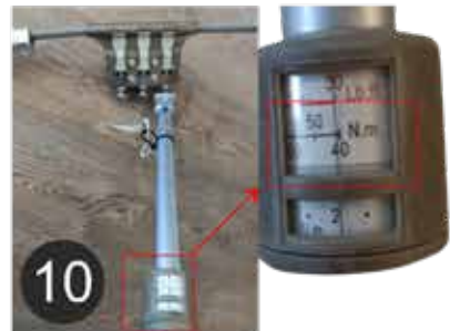
10 Checking the tightness of the M10 screws in CBS Anchors (= 40 N*m).
