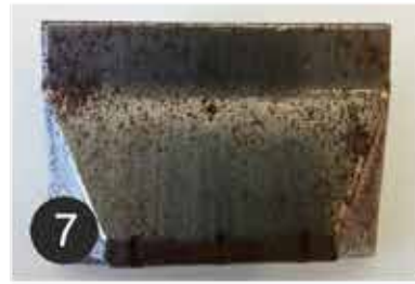
7 Corrosion check on MCD components.
